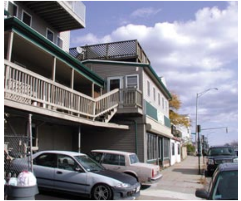
THE LYNNWAY NEAR NEWHALL STREET - BEFORE
